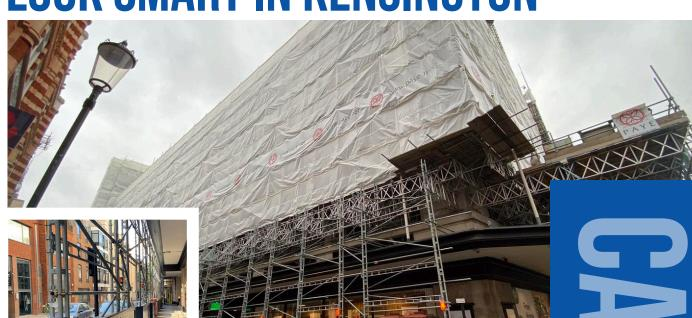
Working closely with UK System Scaffold Hire, JDC Scaffolding developed an innovative gantry design which used HAKI Tripods to minimise disruption in Kensington High Street.
