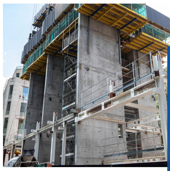
Two 60 metre tall Haki compact stair towers proved the perfect fit when Keltbray undertook the preparatory demolition work for the construction of the Edenica office building in Central London.
