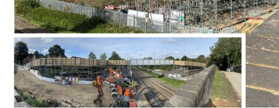
SYS (Scaffolding Contractors) Ltd and UK System Scaffold Hire's collaboration to build a temporary footbridge at Kibworth in Leicestershire is the latest example of the two companies working together to optimise the benefits of the Haki Bridge System - and this time featured two 100 metre long access ramps rather than public access staircases.
