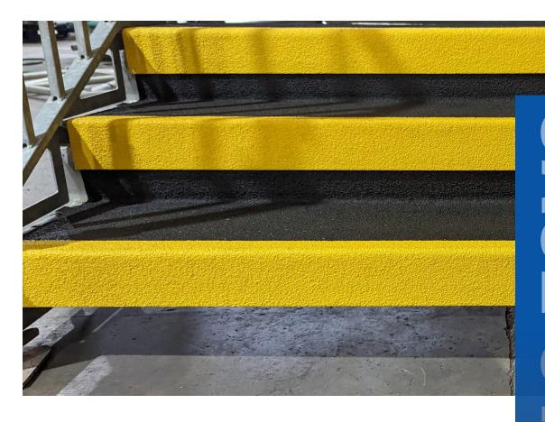
UKSSH has been at the forefront of supplying fully compliant public access staircases for over a decade, with a range of step options including solid treads, enclosed backs and GRP (non-slip) treads.
